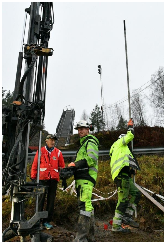
Fjelbolter settes ned i borehullene
