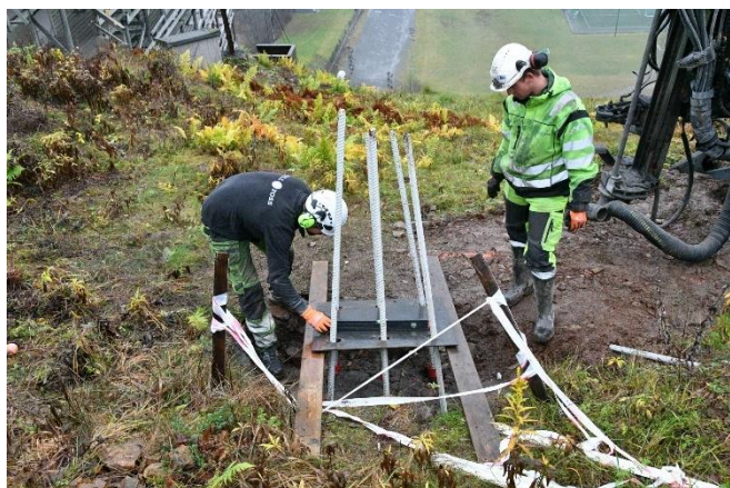
Bergbolter settes ned i borehullene opp ned for å kappes
